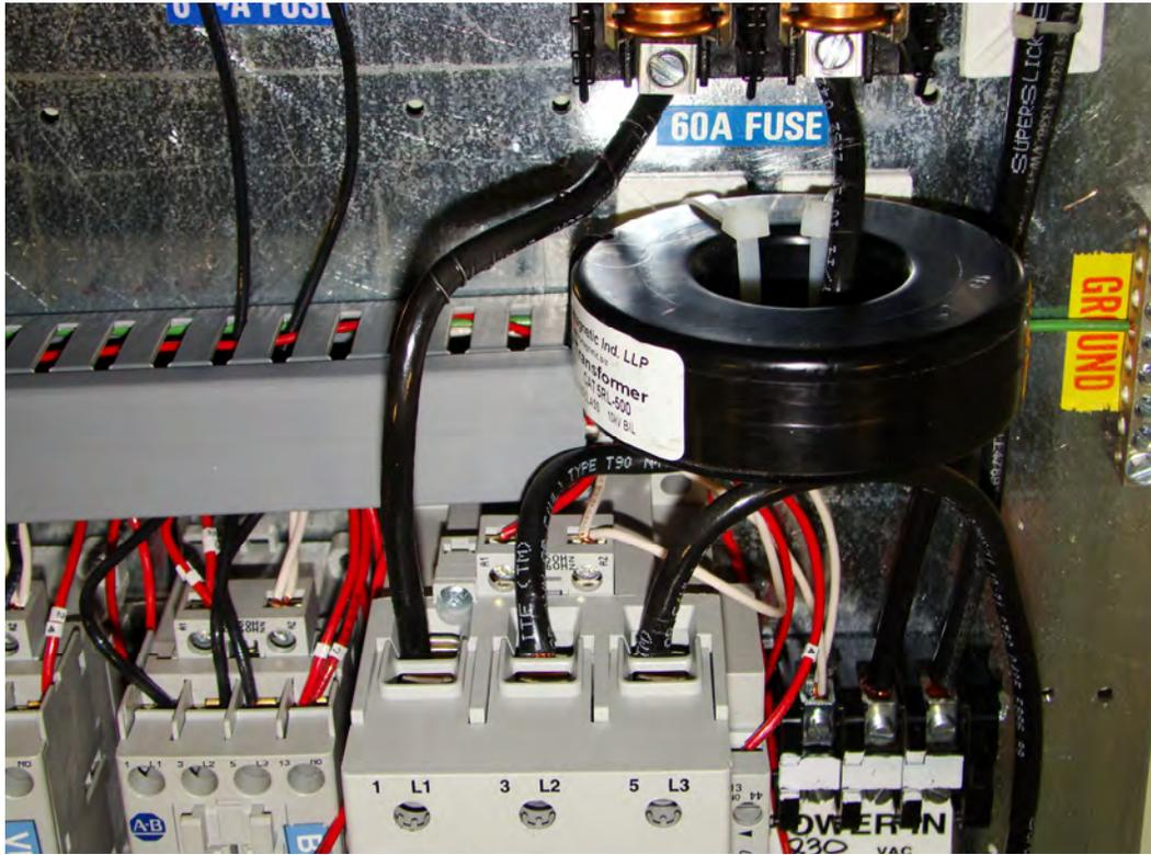
6. Run wires from transformer through wire ways and connect to new meter. Polarity does not matter.
